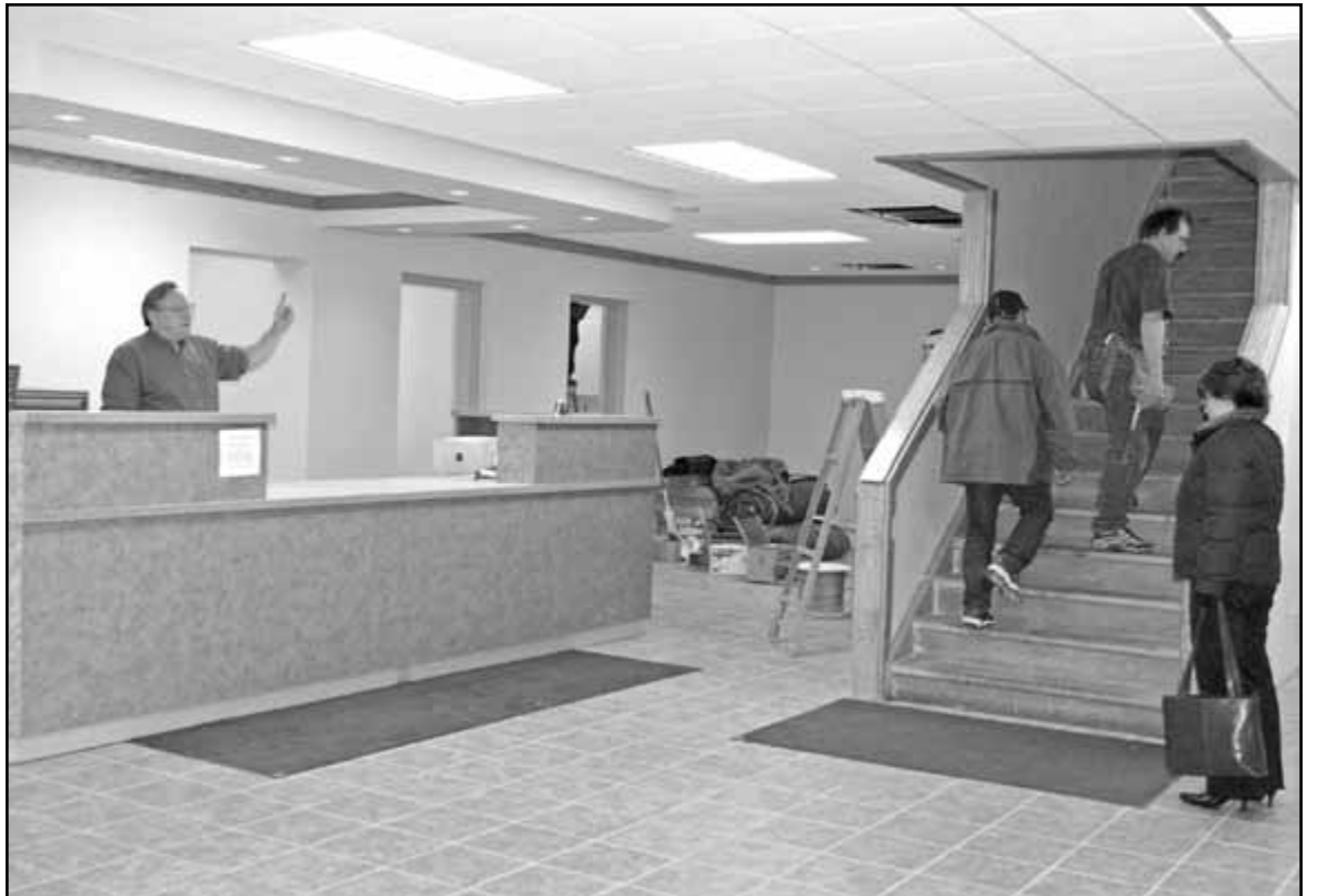
Renovations are underway in the La Ronge Motor Hotel lobby.
