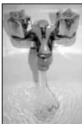
Clean water will soon be flowing from the taps in more on-reserve homes in the La Ronge area, thanks to a new regional management approach and an infusion of federal dollars.
